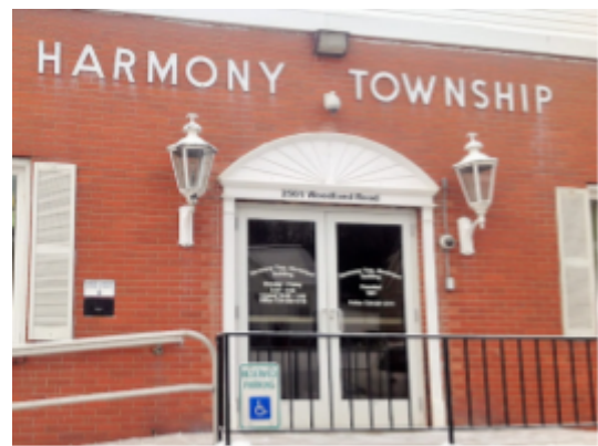
Harmony Township Planning Commission Office 2
